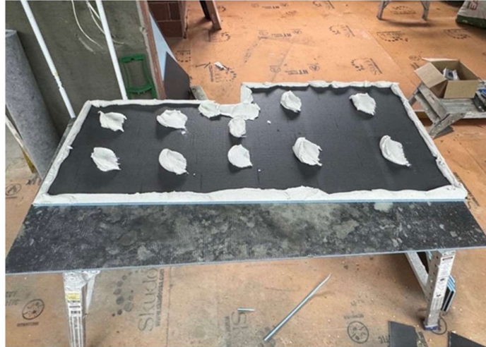
Dot-and-dab adhesive pattern with continuous edge coverage
