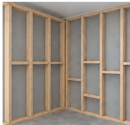
Timber stud wall prior to fixing ThermaSheet
