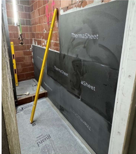
Boards installed to masonry wall
