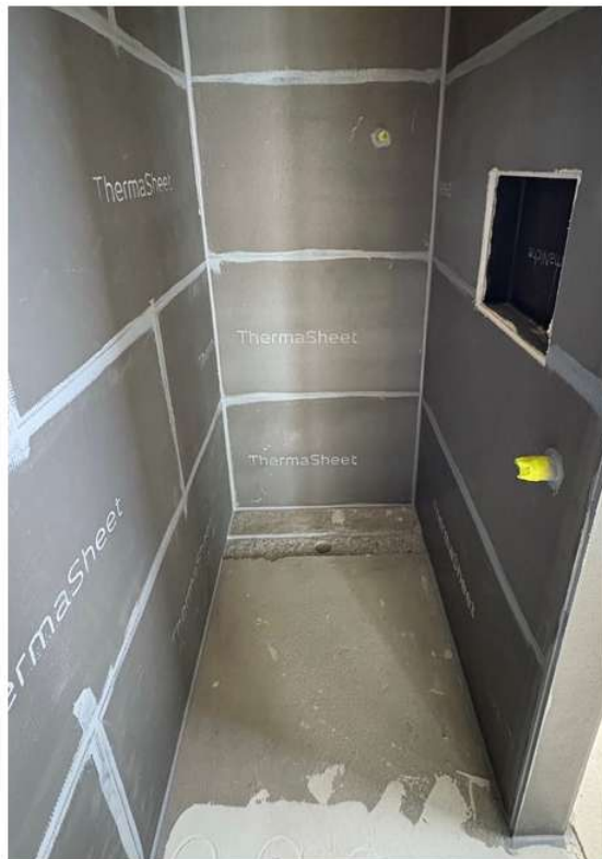
Joint treatment to a ThermaSheet-lined shower area
