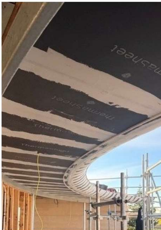
Full mesh render system over 20 mm Thermasheet board
