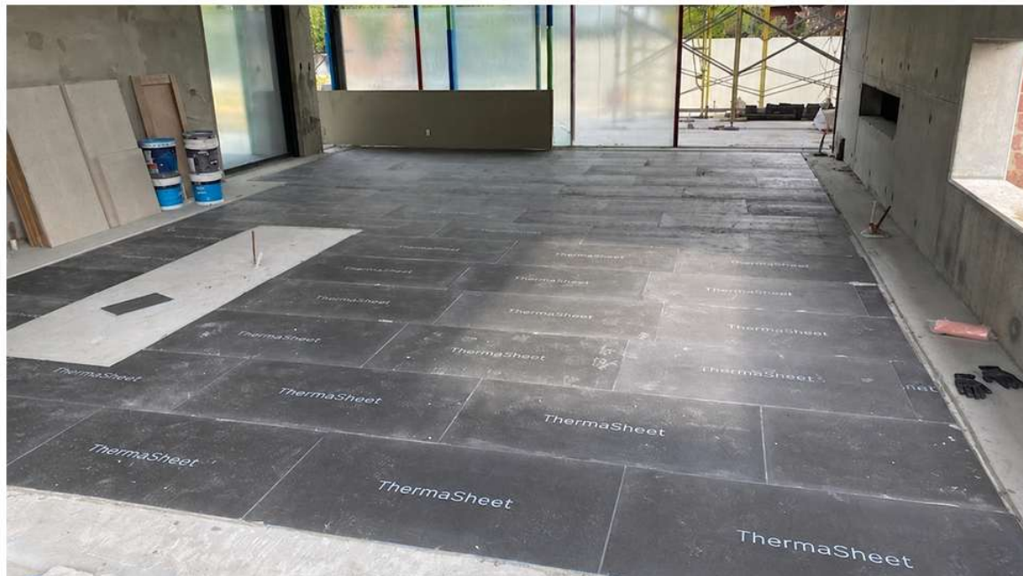
Thermasheet floor-fixed boards installed over a prepared floor
